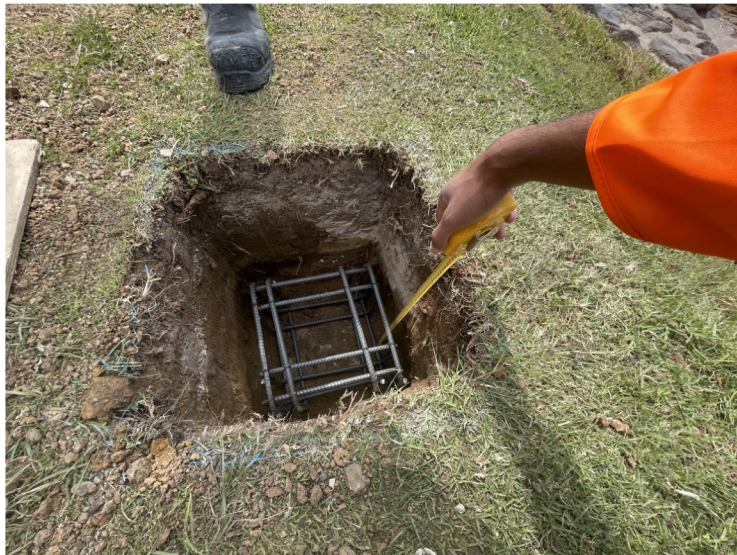
Figure 4: Hole only 600mm deep
