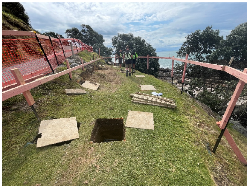
Figure 1: Overview of Site
